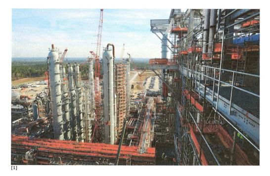
GASIFIER: Kemper's gasifier unit is designed to convert lignite coal into synthesis gas, which can be burned in the facility's turbines to generate electricity.
